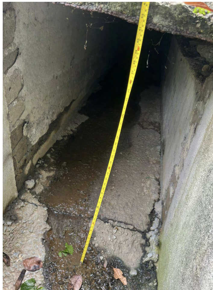
Dimension of 1000mm Box Culvert
