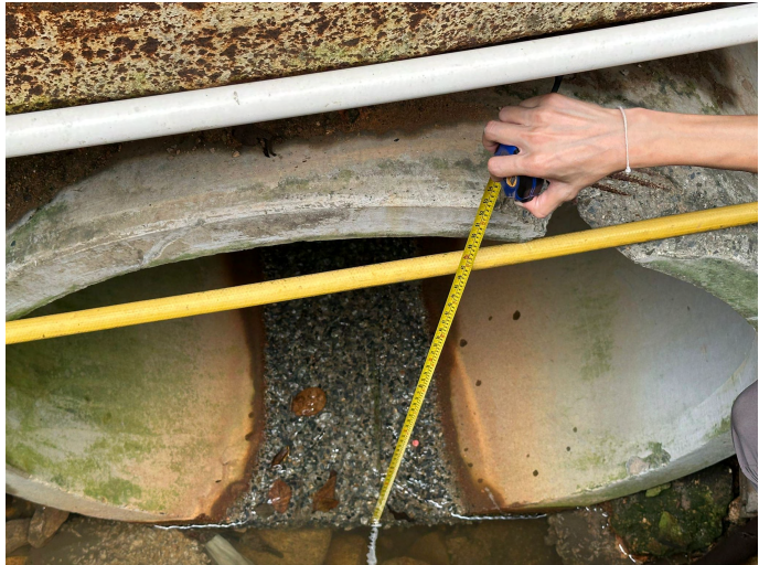
SITE PHOTO 6 EXISTING UNDERGROUND 1000mm dia. PIPE
