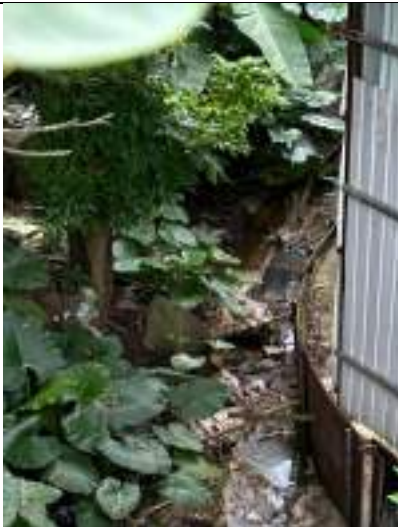
Site Photo 1c: Stepped Channel and Existing Stream (3m (W) x2m(H))
