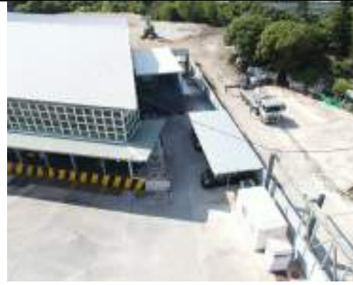
Aerial Photo 6: Site Entrance
