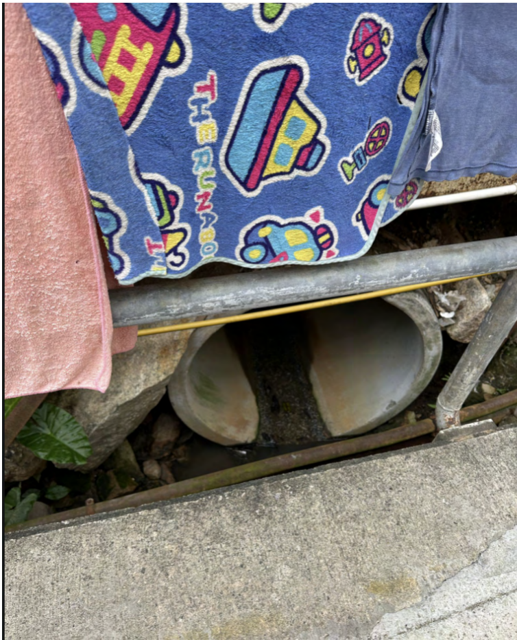
SITE PHOTO 6 EXISTING UNDERGROUND 1000mm dia. PIPE
